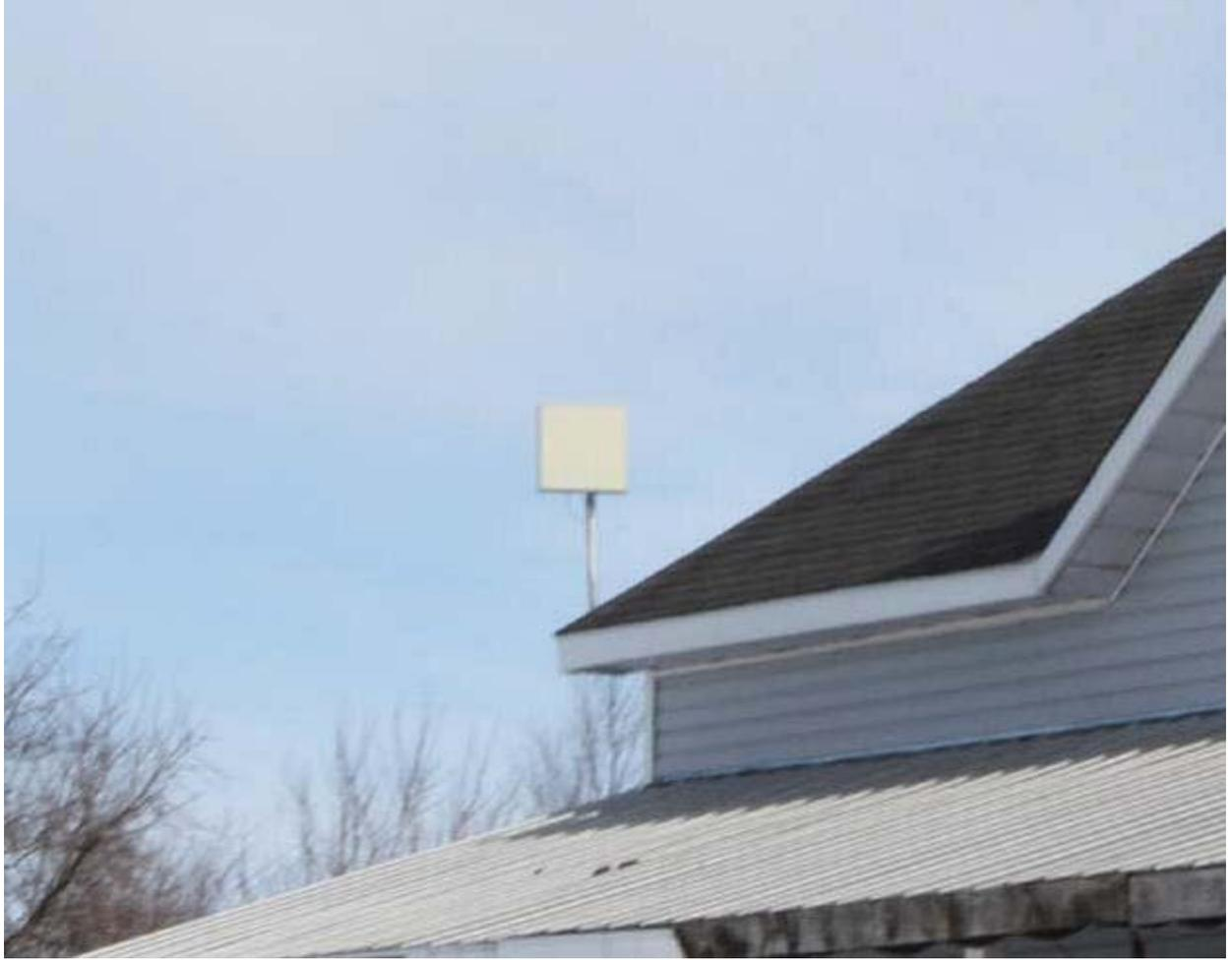
Diagram 3 Roof Mounted Antenna
