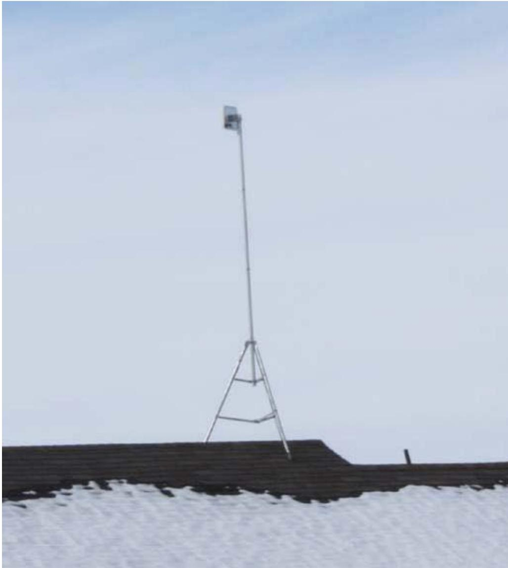
Diagram 4 Roof Tripod Mounted Antenna
