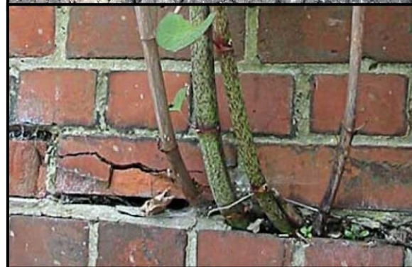
Japanese knotweed can grow through 8cm of concrete/asphalt (top) and impact foundations and walls (below).
