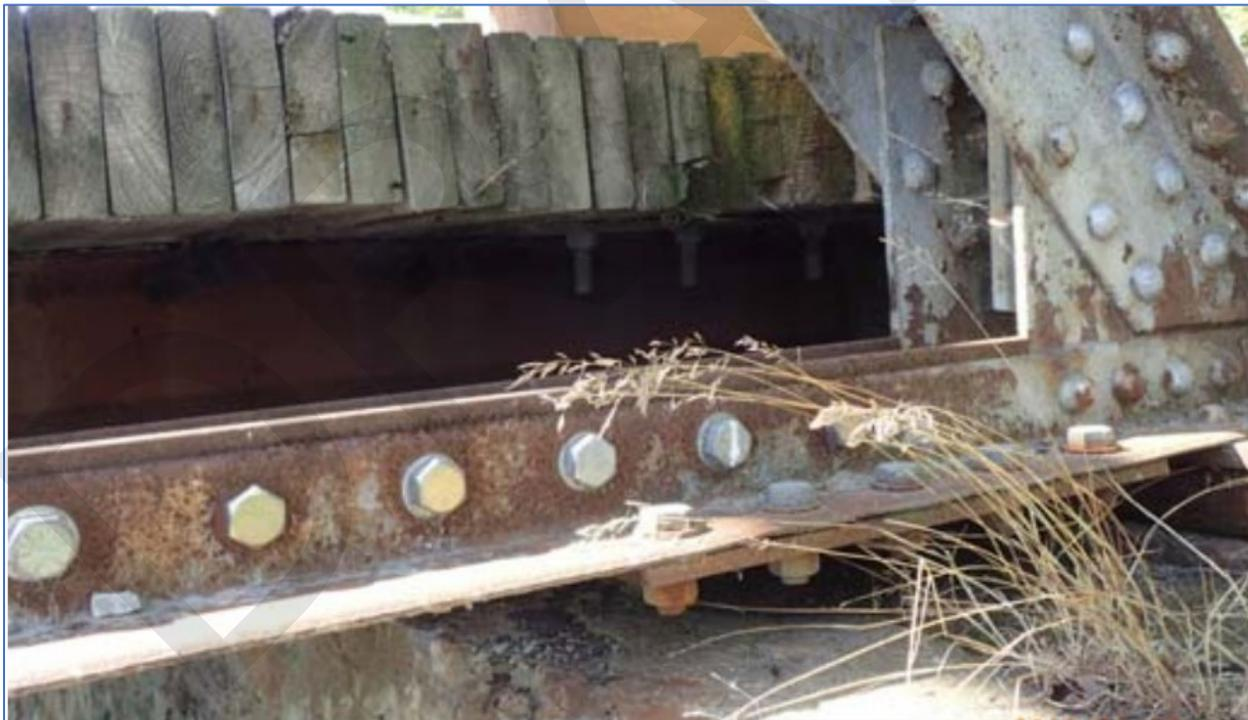
Figure 27: View of bolted stringer ends.<sup>141</sup>
