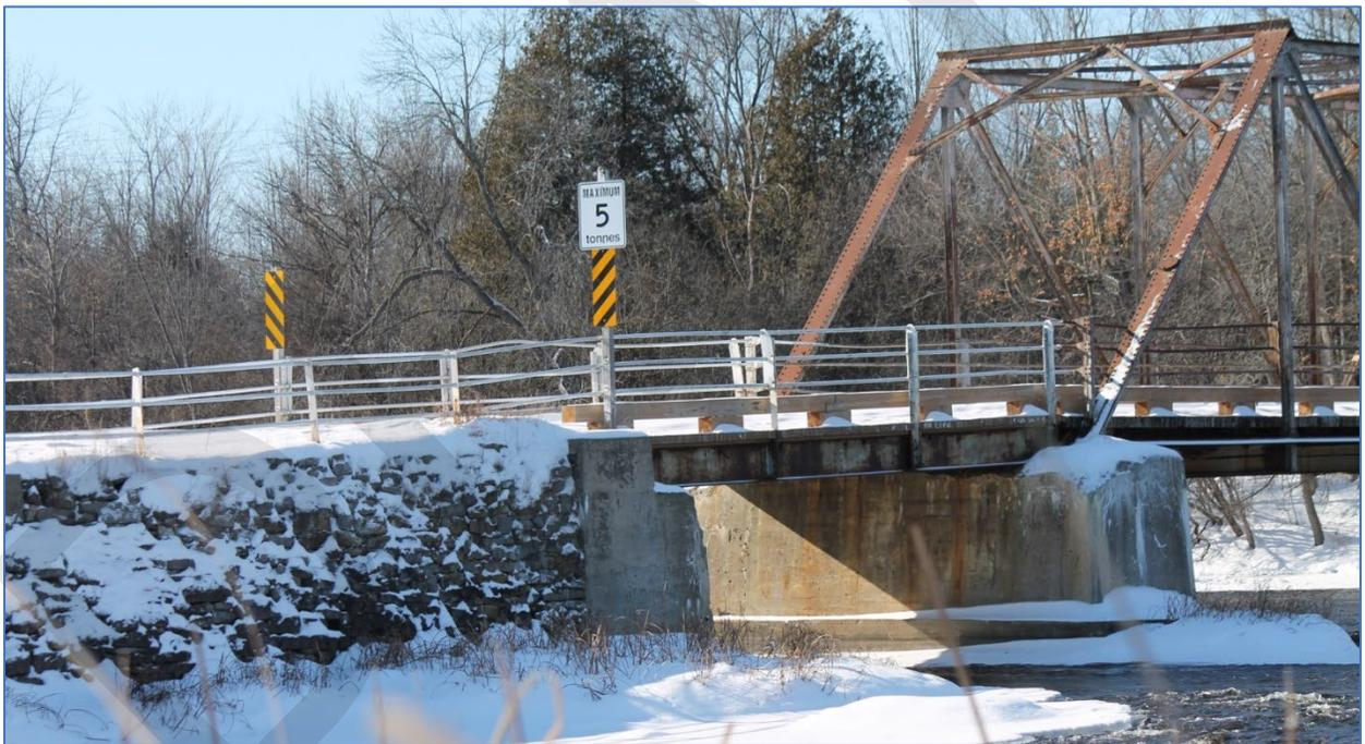
Figure 33: View of dry-stone retaining wall, pier, and 9.2 m span.
