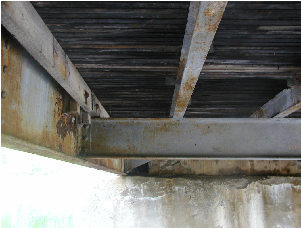
Photograph 17: Configuration of below-deck structural steel in slab-on-girder span.
