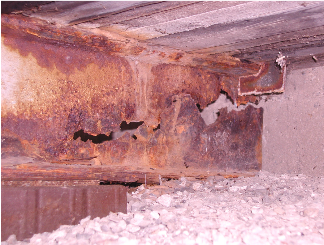
Photograph 19: Very severe section loss in web of middle stringer, West Abutment.
