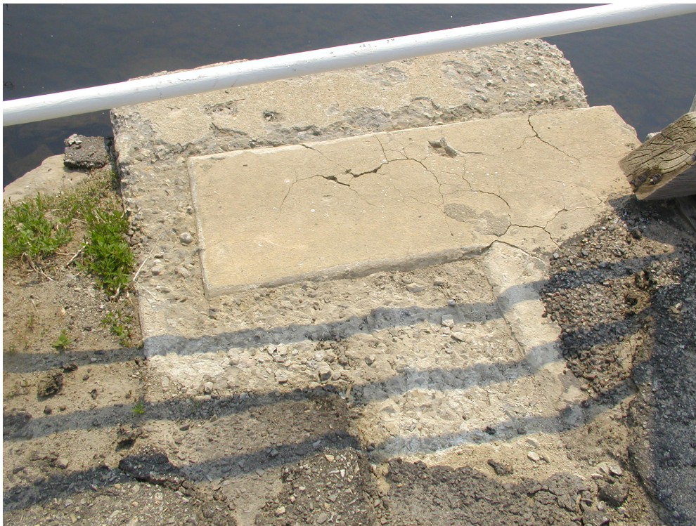
Photograph 32: Detail of top of East Abutment, showing concrete encasement. West Abutment similar.
