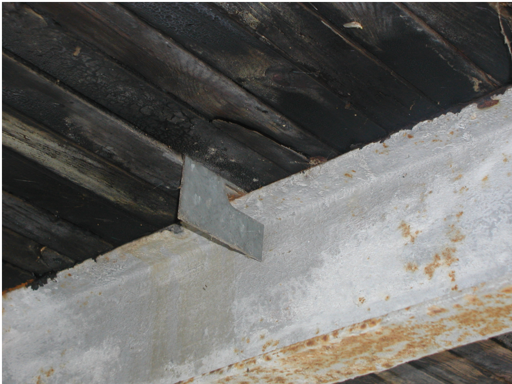
Photograph 18: Detail of clip attaching deck to stringer,
