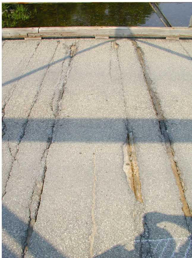
Photograph 8: Detail of asphalt deterioration on timber deck.
