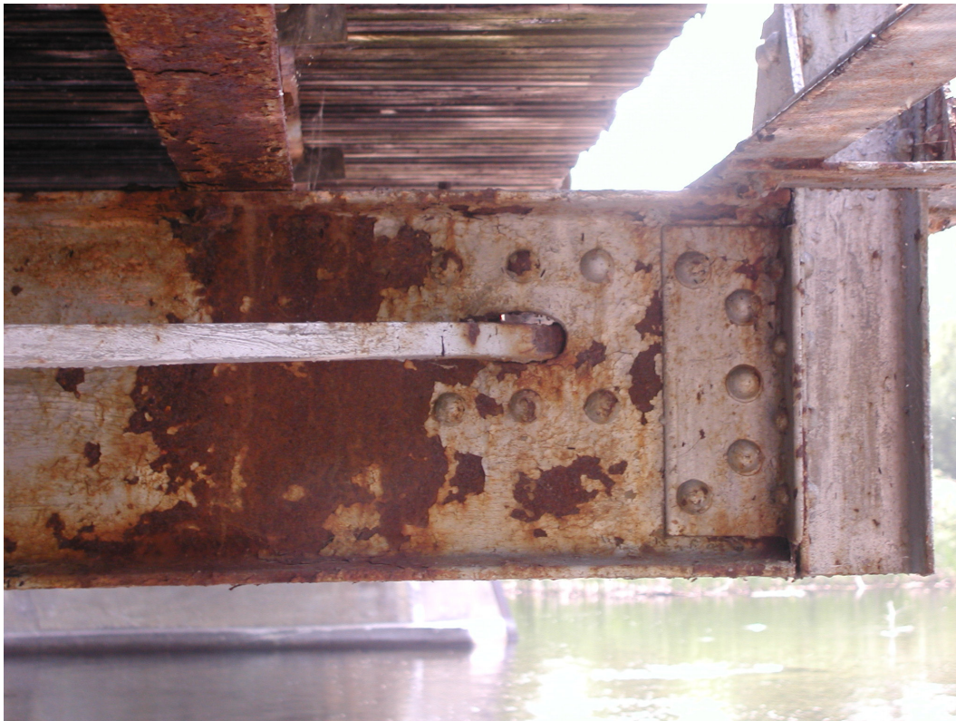
Photograph 15: Detail of cross-bracing as it passes through the web of the floorbeam.
