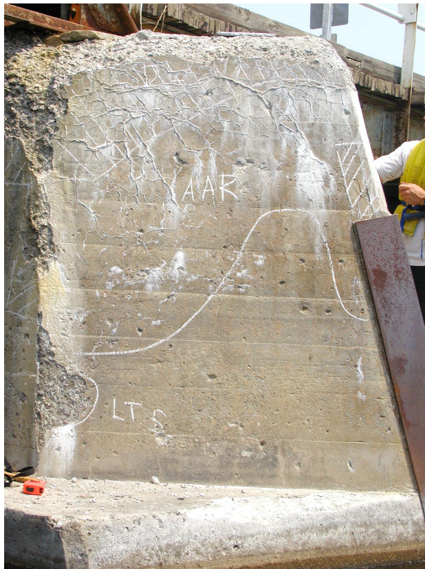
Photograph 28: Deterioration of west face of pier nosing. Note extensive deterioration and alkali-aggregate reaction. Condition of east face is similar.
