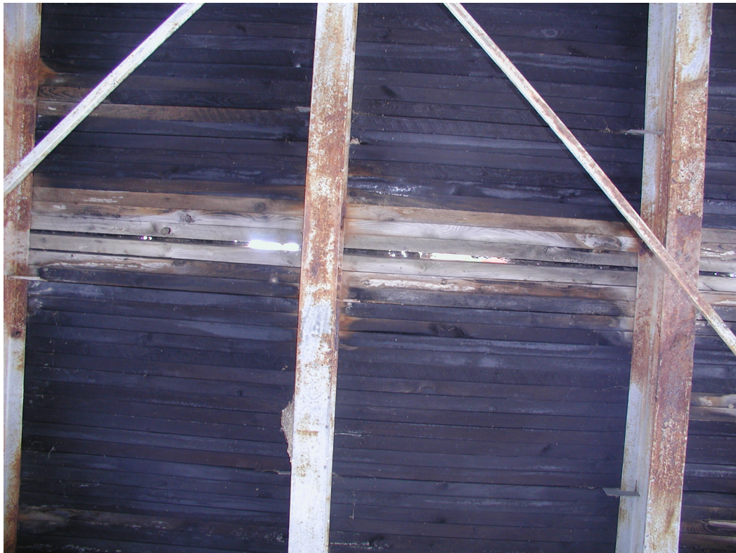
Photograph 12: Creosote is generally missing on timbers in locations of gaps, which have allowed penetration of water.
