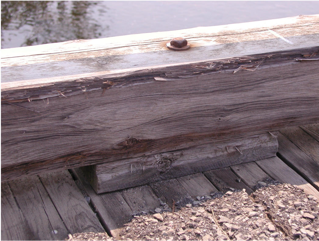
Photograph 33: Detail of curb on timber deck.
