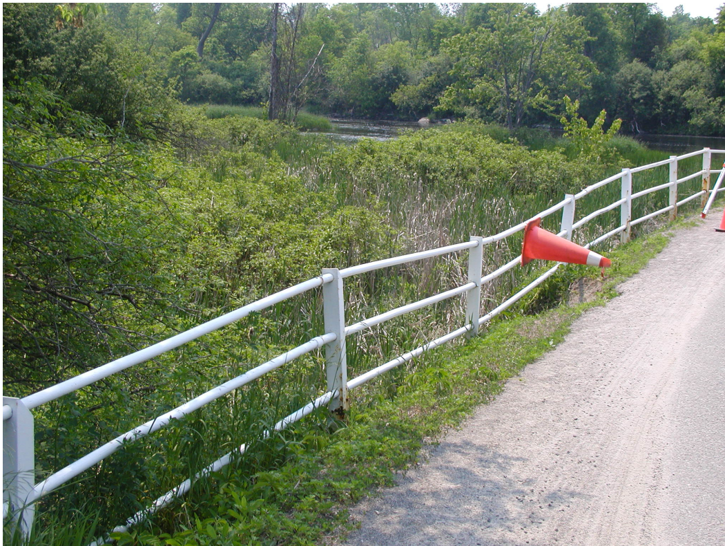
Photograph 34: Deformed railing on south side of east approach retaining wall as a result of slope erosion undermining posts.
