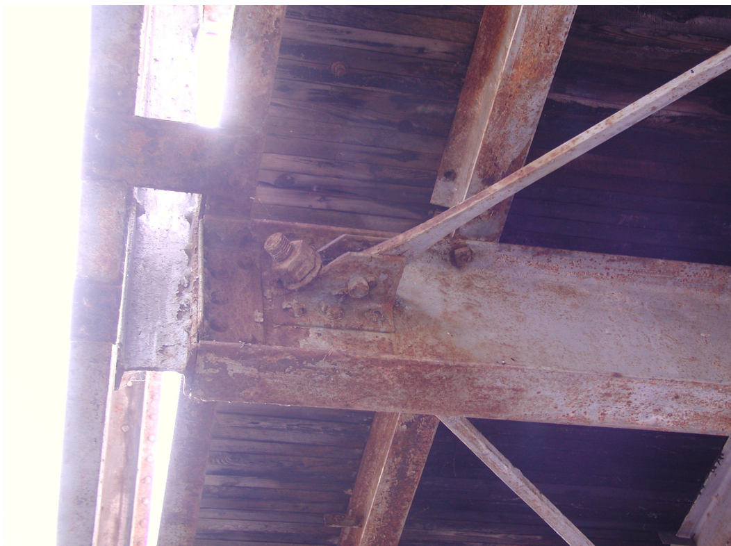
Photograph 16: Detail of cross-bracing connection at floorbeam.
