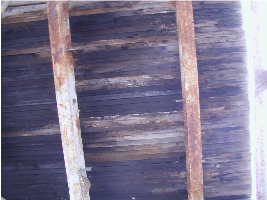
Photograph 11: Exterior stringers typically exhibit more corrosion than interior stringers.
