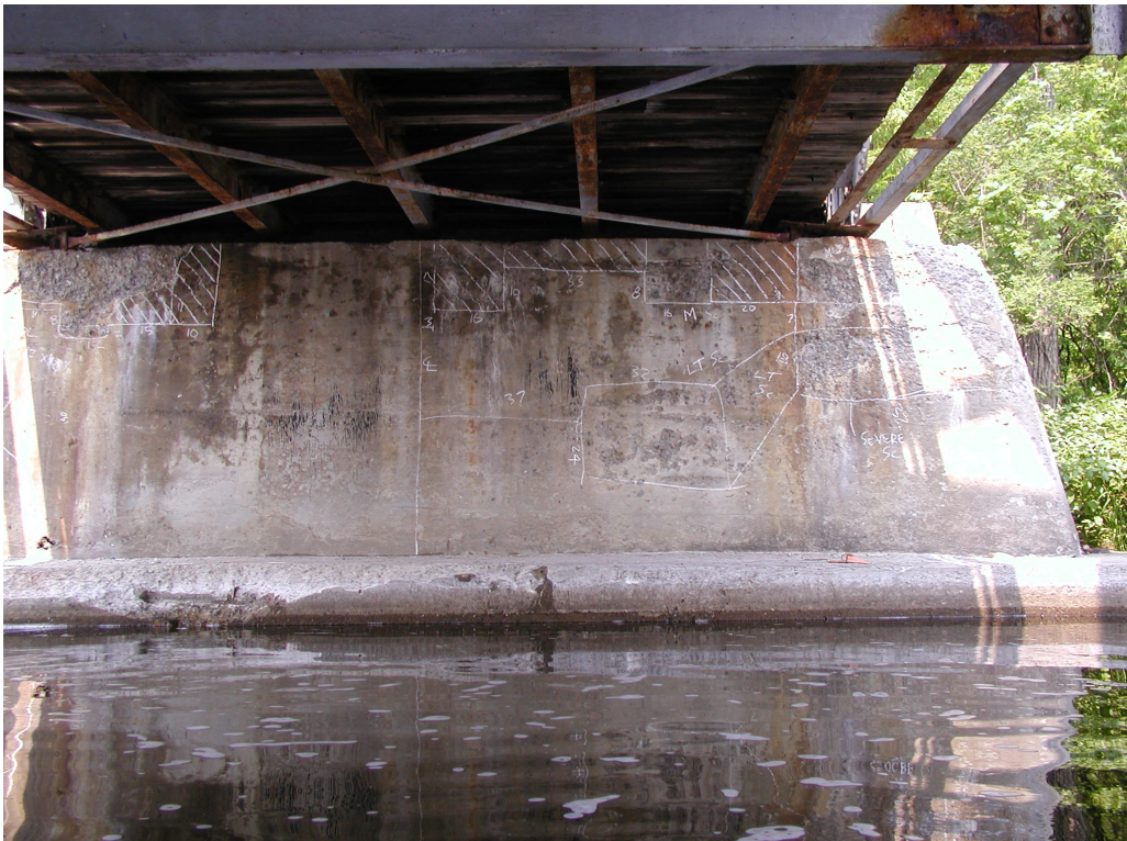
Photograph 26: Face of West Abutment is characterized by extensive scaling, delaminations, and alkali-aggregate reaction. Condition of face of East Abutment is similar.
