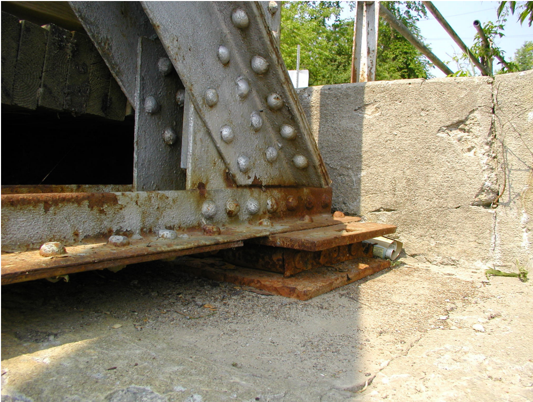
Photograph 21: Bearing configuration at West Abutment.
