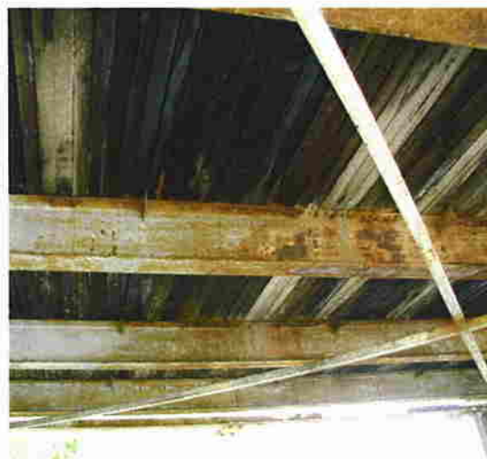
Photograph 5: Deterioration of the timber deck due to loss of creosote protection. Note the widespread light corrosion of the below-deck steel floor system.
