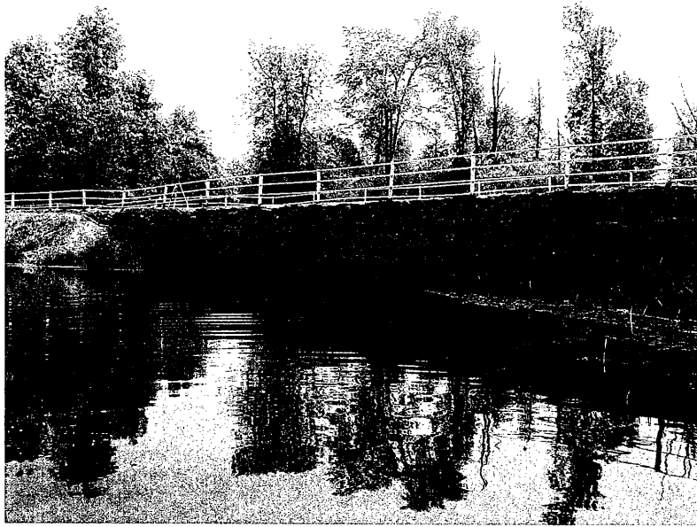
Photograph 5: Dry stone retaining wall on east approach.
