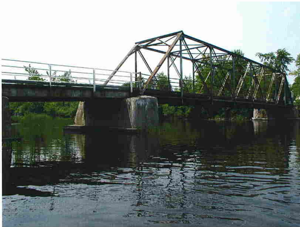
Photograph 1: North elevation of Andrewsville Bridges, showing truss and slab on girder spans.
