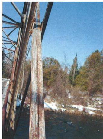
Photograph 7: Buckling of U4L3' (east truss) near mid-height.
