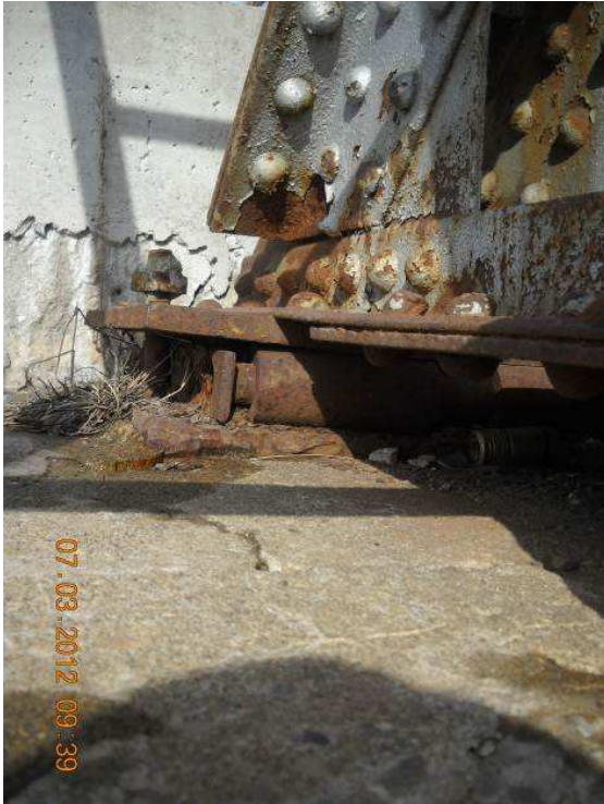
Photograph 8: Condition of truss bearing. Southeast bearing shown.
