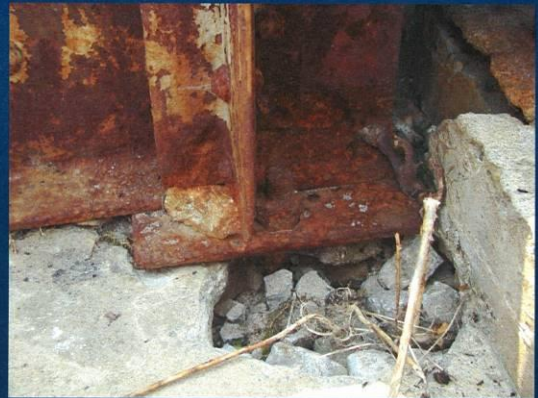
Undermining of south pier bearing
