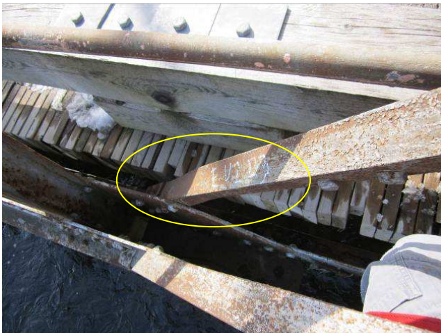
Photograph 6: Twisting of U2L3 (east truss) near L3.
