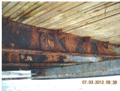
Photograph 2: Typical stringer corrosion in end bay of truss span.
