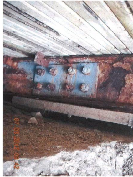
Photograph 9: Displace timber blocking at stringer bearing. Note stringer web repair from 2009 rehabilitation.
