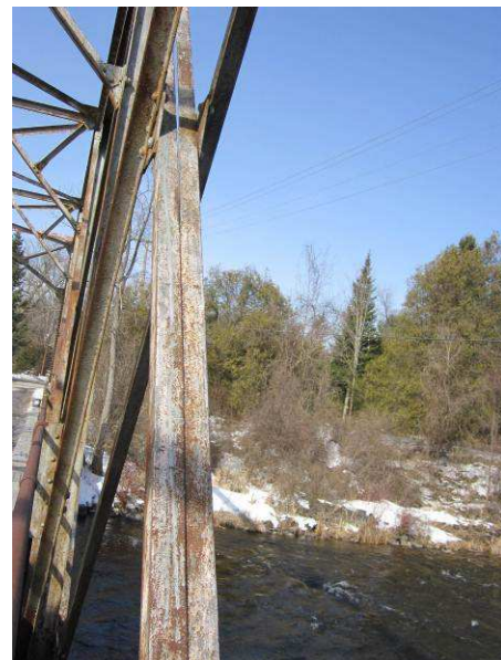
Photograph 7: Buckling of U4L3' (east truss) near mid-height.
