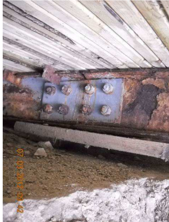
Photograph 9: Displace timber blocking at stringer bearing. Note stringer web repair from 2009 rehabilitation.
