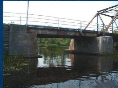
Single span slab-on-girder
