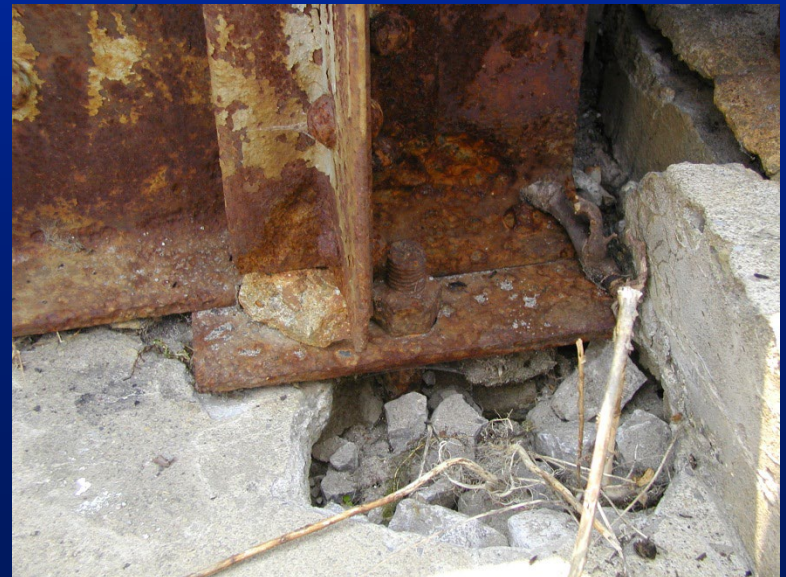
Undermining of south pier bearing
