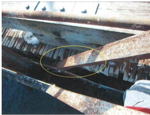
Photograph 6: Twisting of U2L3 (east truss) near L3.
