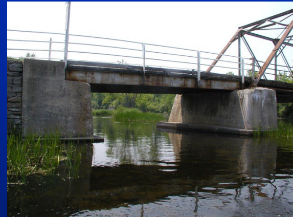
Single span slab-on-girder
