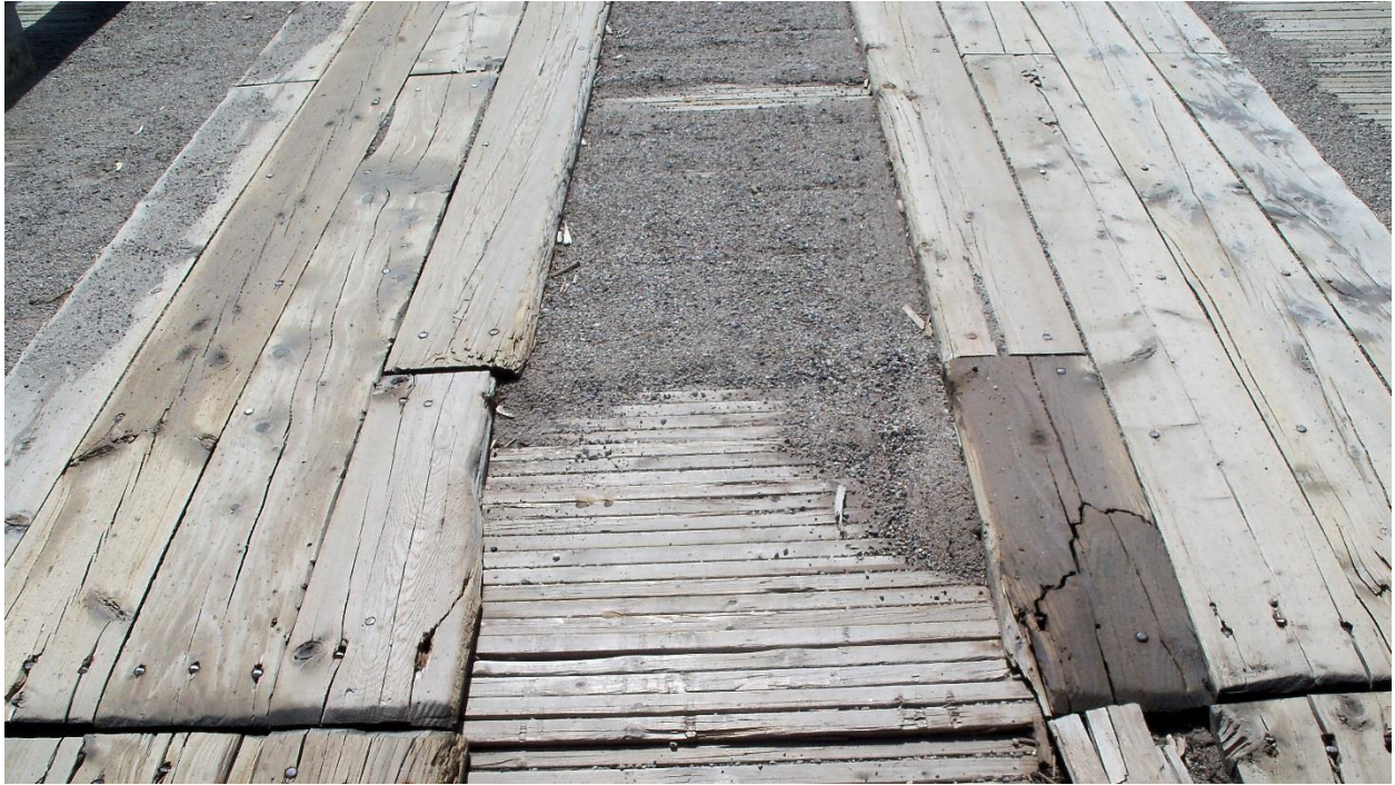
View of deck wearing surface with rot, splits, and checks
