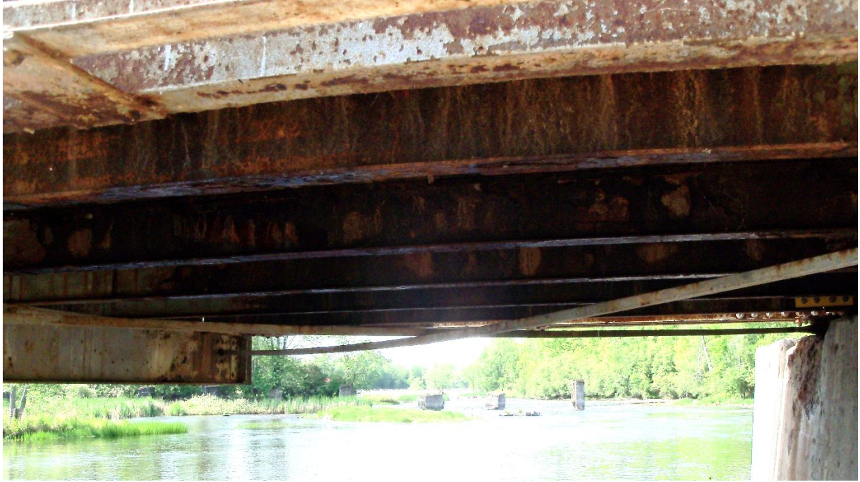
View showing cross bracing and corrosion on girders
