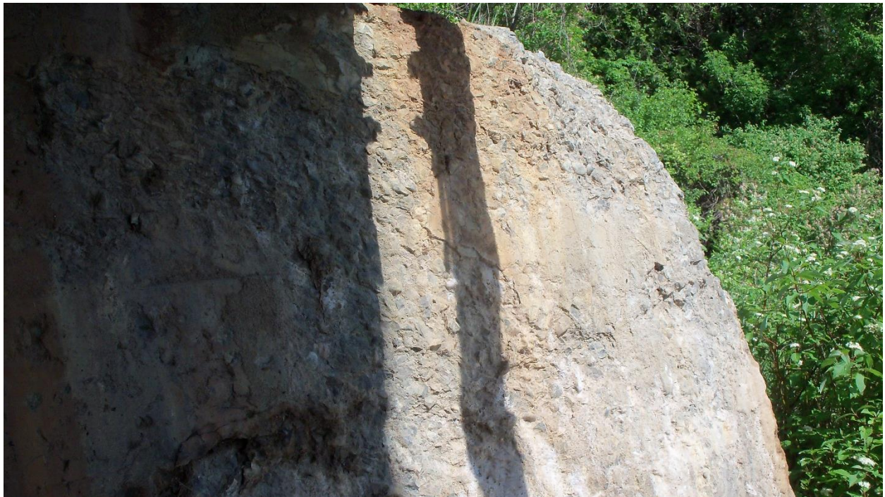
View showing mass spalling and corrosion stains
