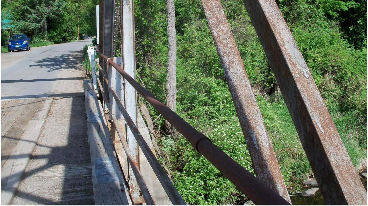
View of timber curb and railing system
