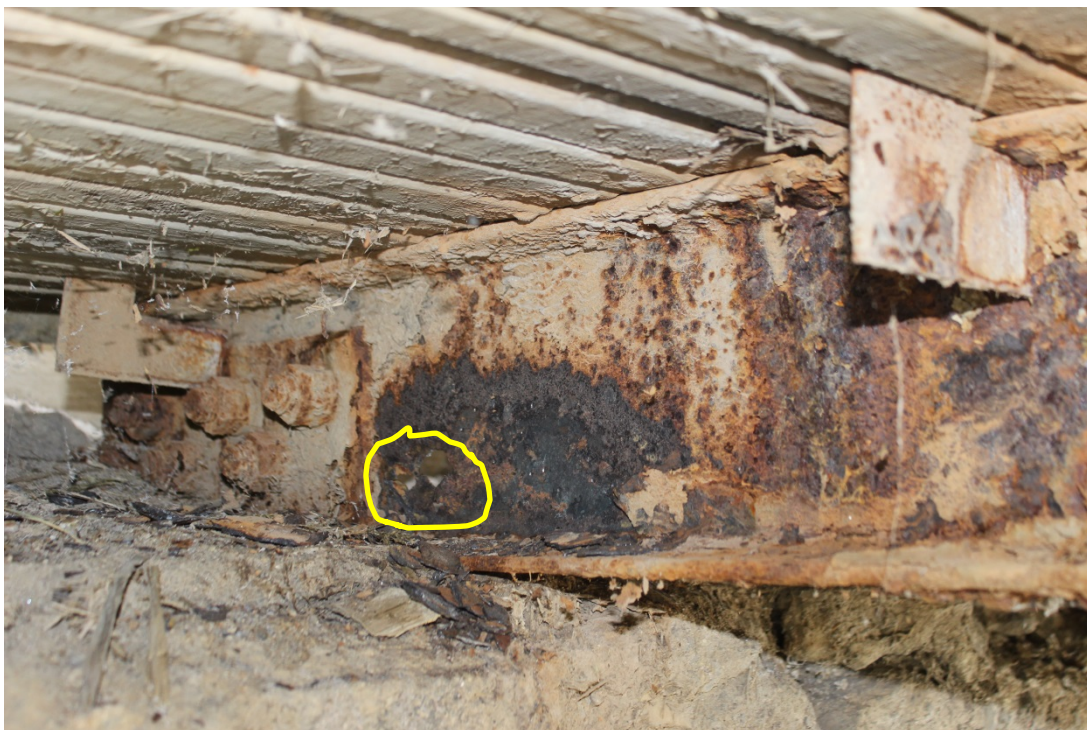
Image 28. Perforated Stringer 2 at east abutment bearing
