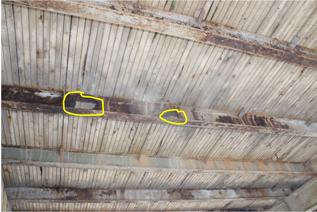
Image 15. General view of west bay of approach span looking downstream. Perforations circled.
