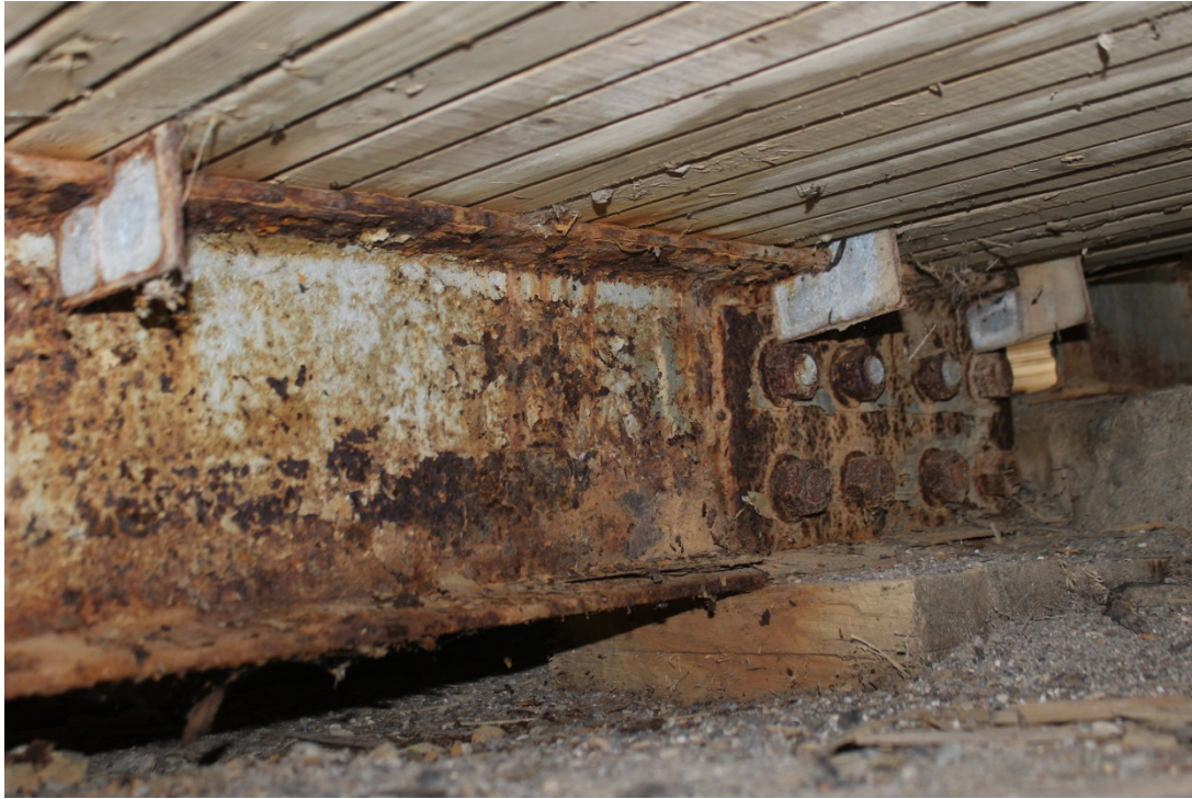
Image 9. Truss Stringer 3 at Pier Bearing
