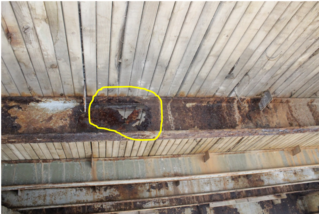
Image 12. Perforation of Approach Stringer 2 before probing
