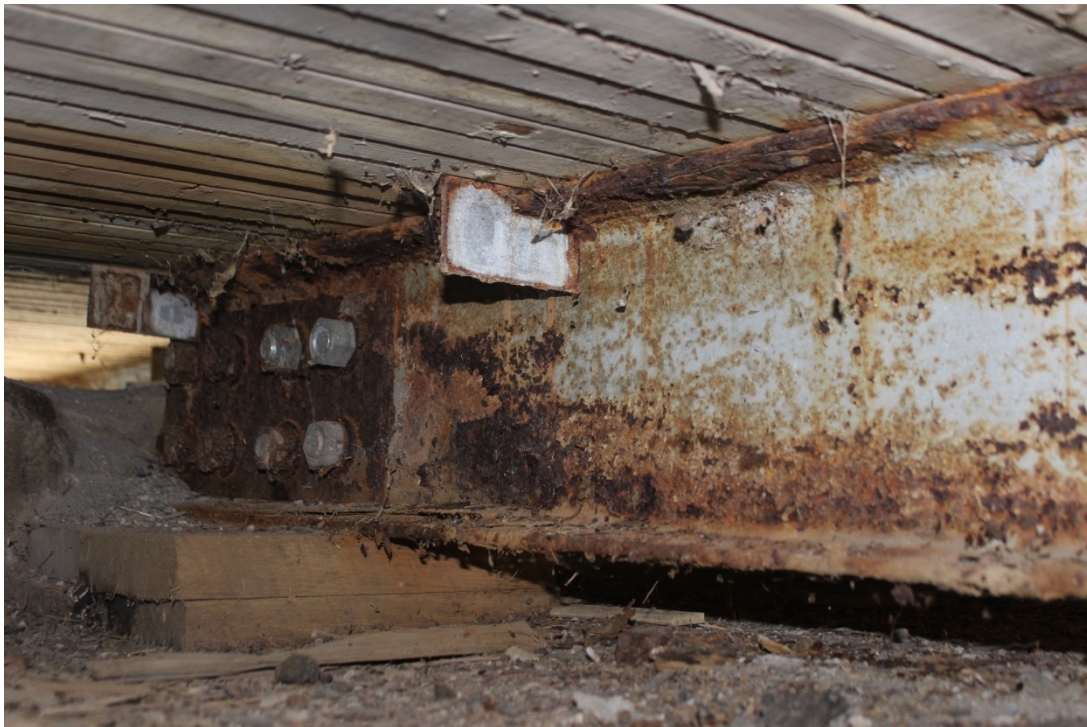
Image 8. Truss Stringer 2 at Pier Bearing
