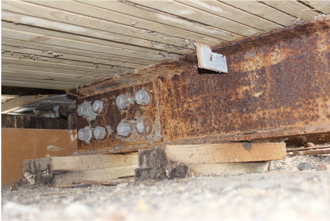
Image 7. Truss Stringer 1 at Pier Bearing
