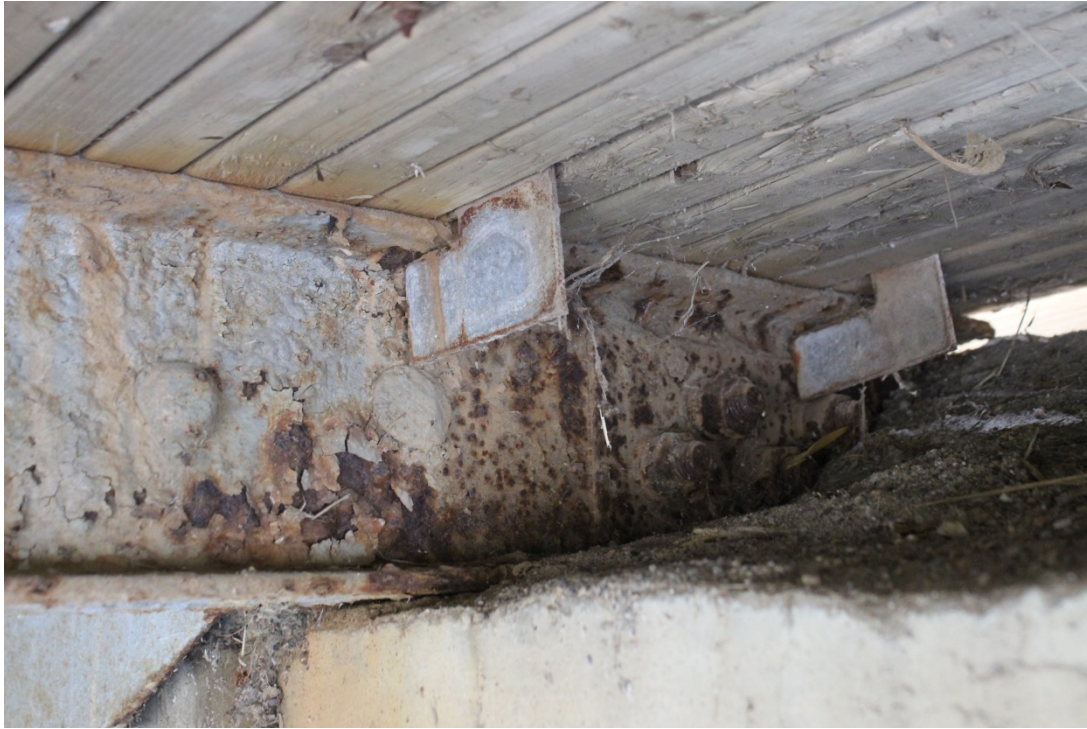
Image 25. Stringer 5 bearing area at east abutment
