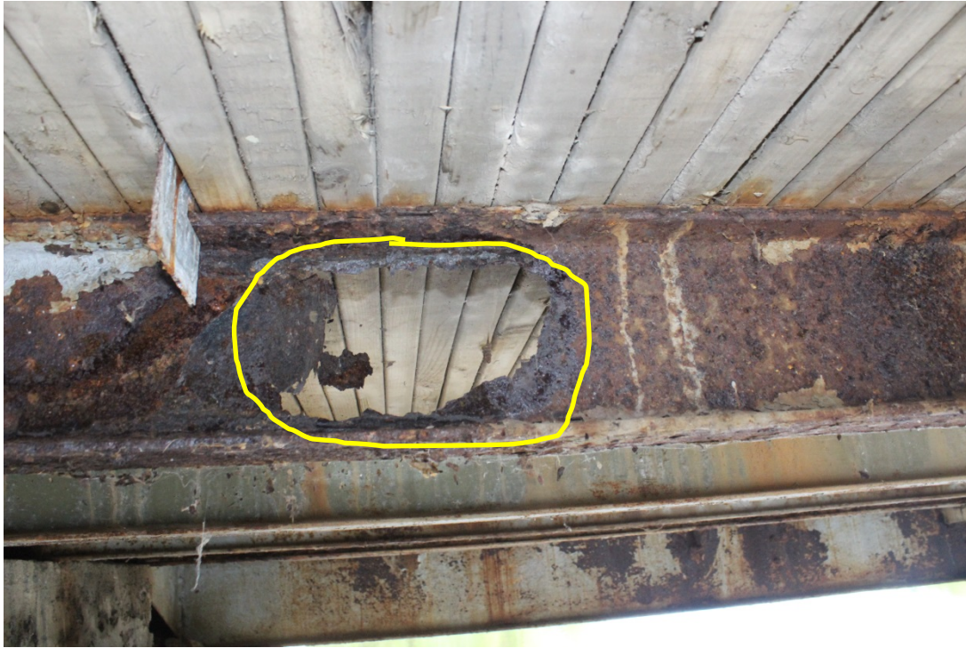
Image 13. Perforation of Approach Stringer 2 after probing
