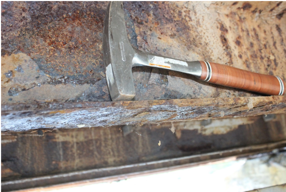
Image 6. Typical corrosion on stringers Bay 1
