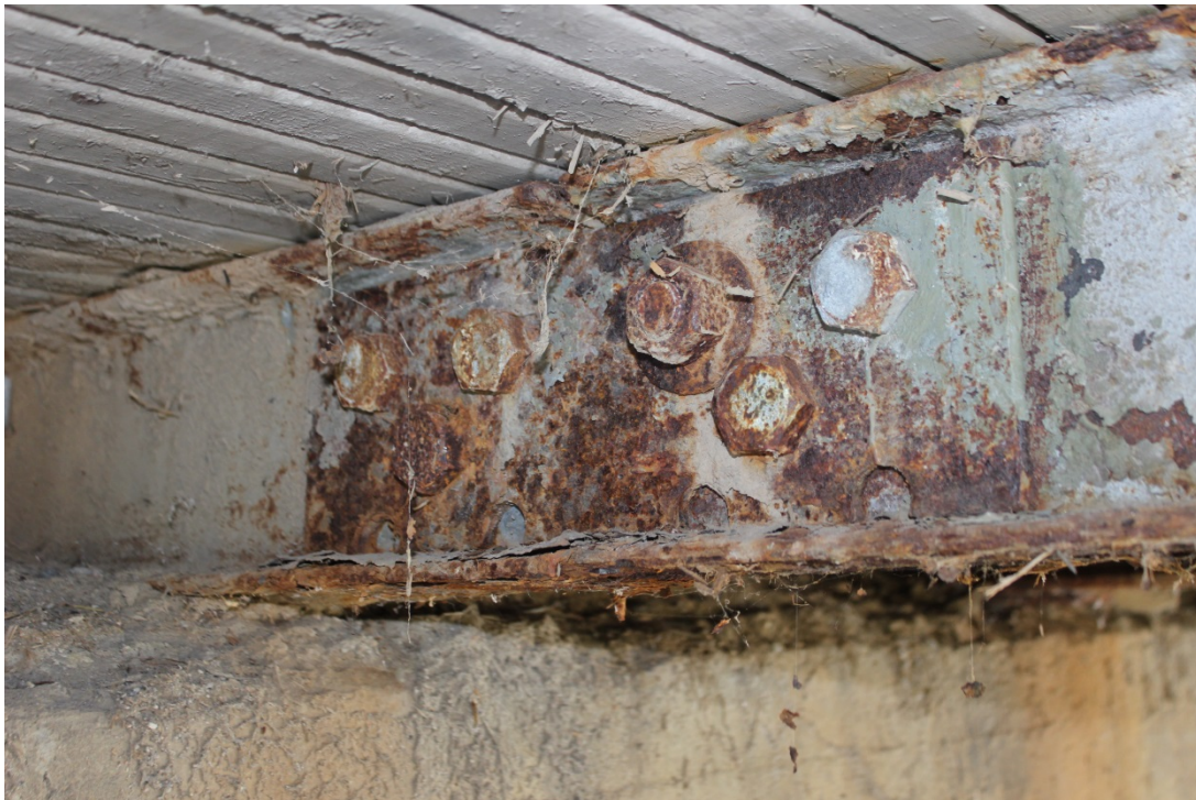
Image 26. Splice on Stringer 4 at east abutment
