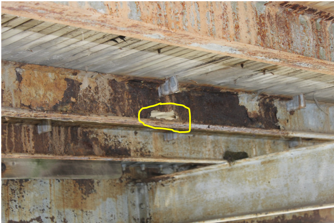
Image 34. Close-up of perforation shown in Image 33
