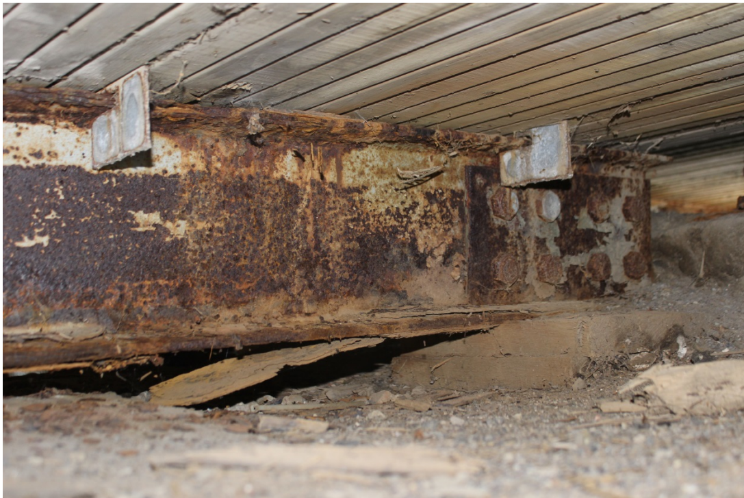
Image 10. Truss Stringer 4 at Pier Bearing
