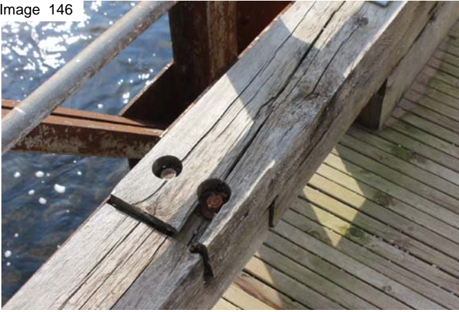
Curb timber decay on truss
