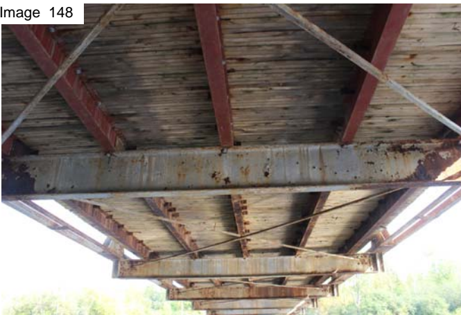
Curb timber decay on truss
