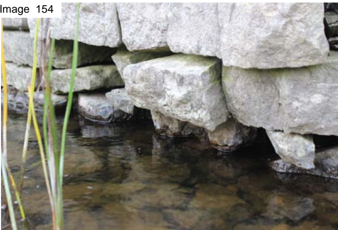
Disintegrating pier nosing
