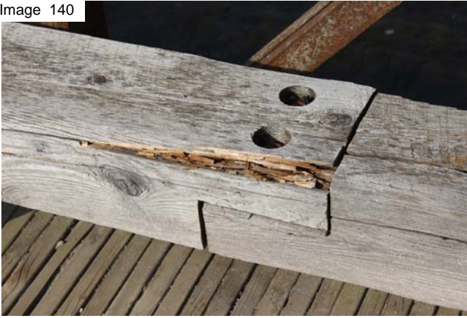
Decay in curb timber
