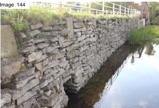
Under-cut rail post foundation SE quadrant
