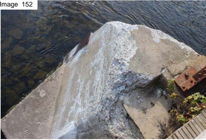
Disintegrating pier nosing
