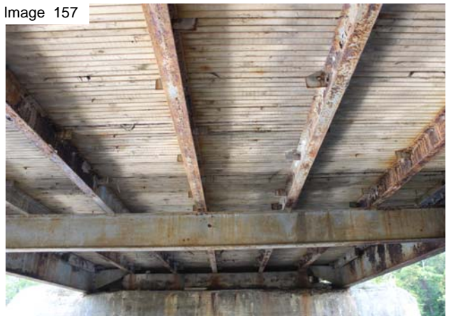
Peforation stringer 2 approach span south end
