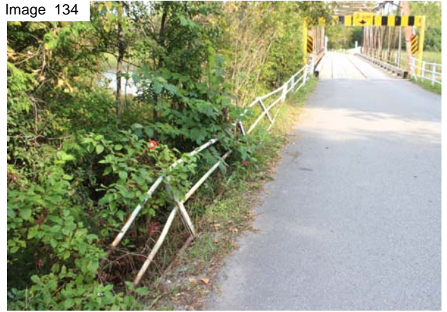
Damaged pipe railing NE quadrant
