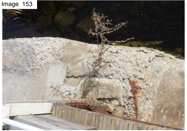
Disintegrating south abutment west side
