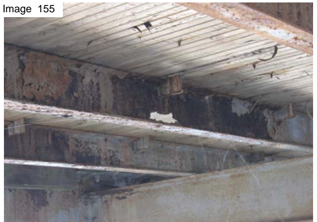
Disintegrating south abutment west side
