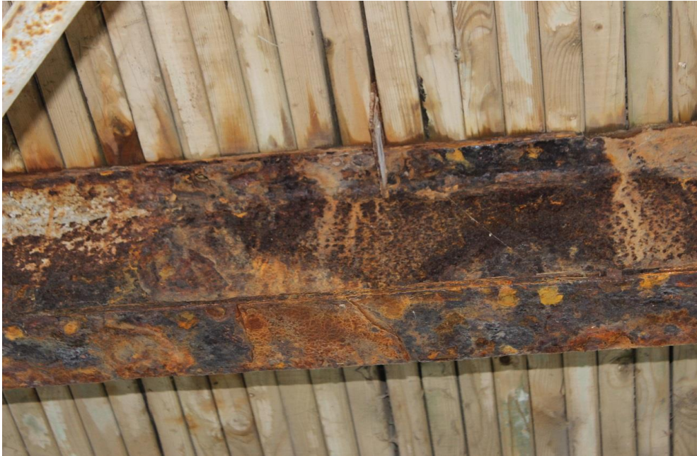
Image 9. South face of Stringer 3 between FB 7 & pier, slab rust and general section loss
