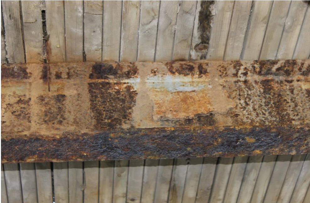
Image 3. Stringer 4 north side adjacent FB 2, slab rust, severe corrosion
