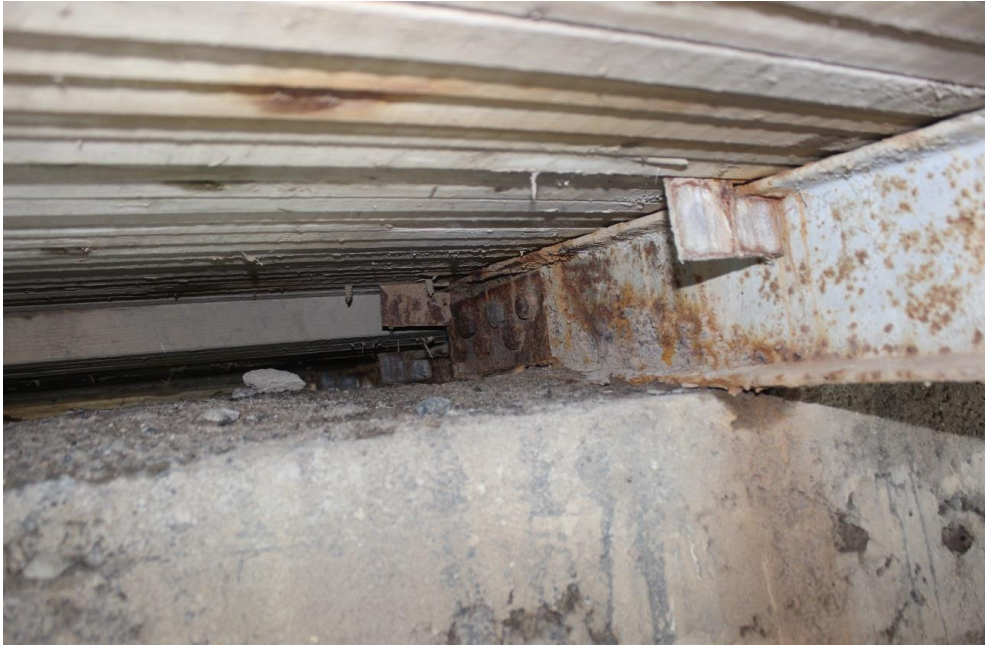
Image 17. Approach span stringer resting on east abutment
