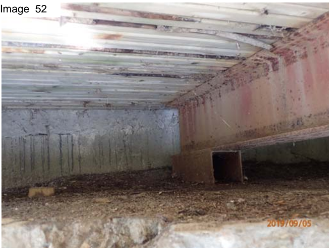
West end ballast wall & stringer
