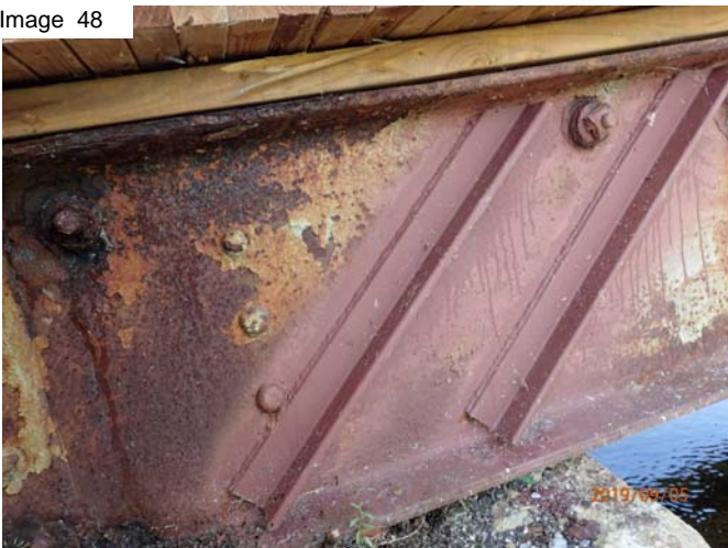
SE girder end web strengthening (2019)
