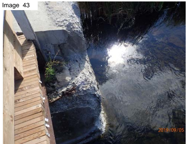
South abutment west corner disintegration
