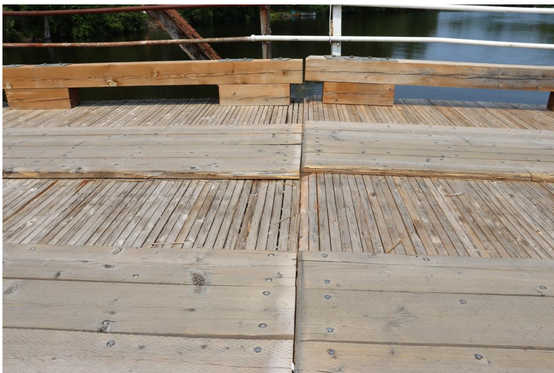
Figure 54: Grade change / bump over pier
