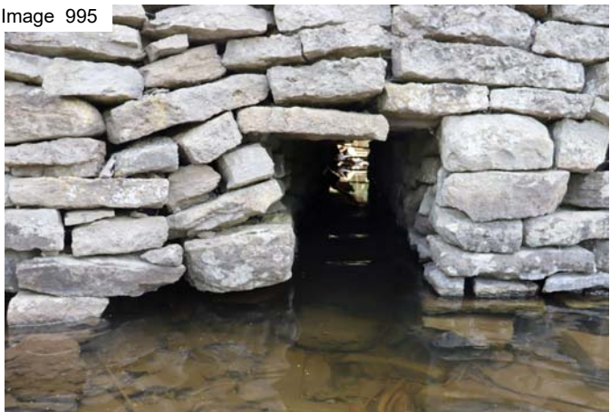
Culvert through causeway
