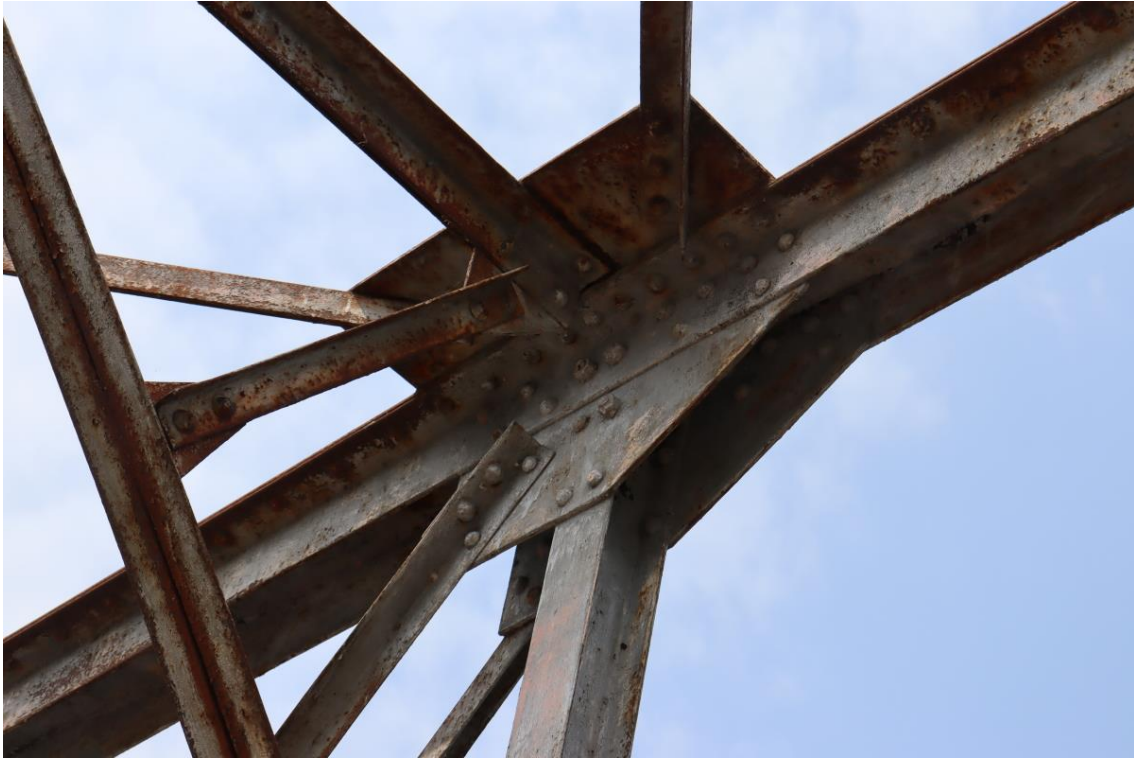
Figure 57: Typical top chord connection
