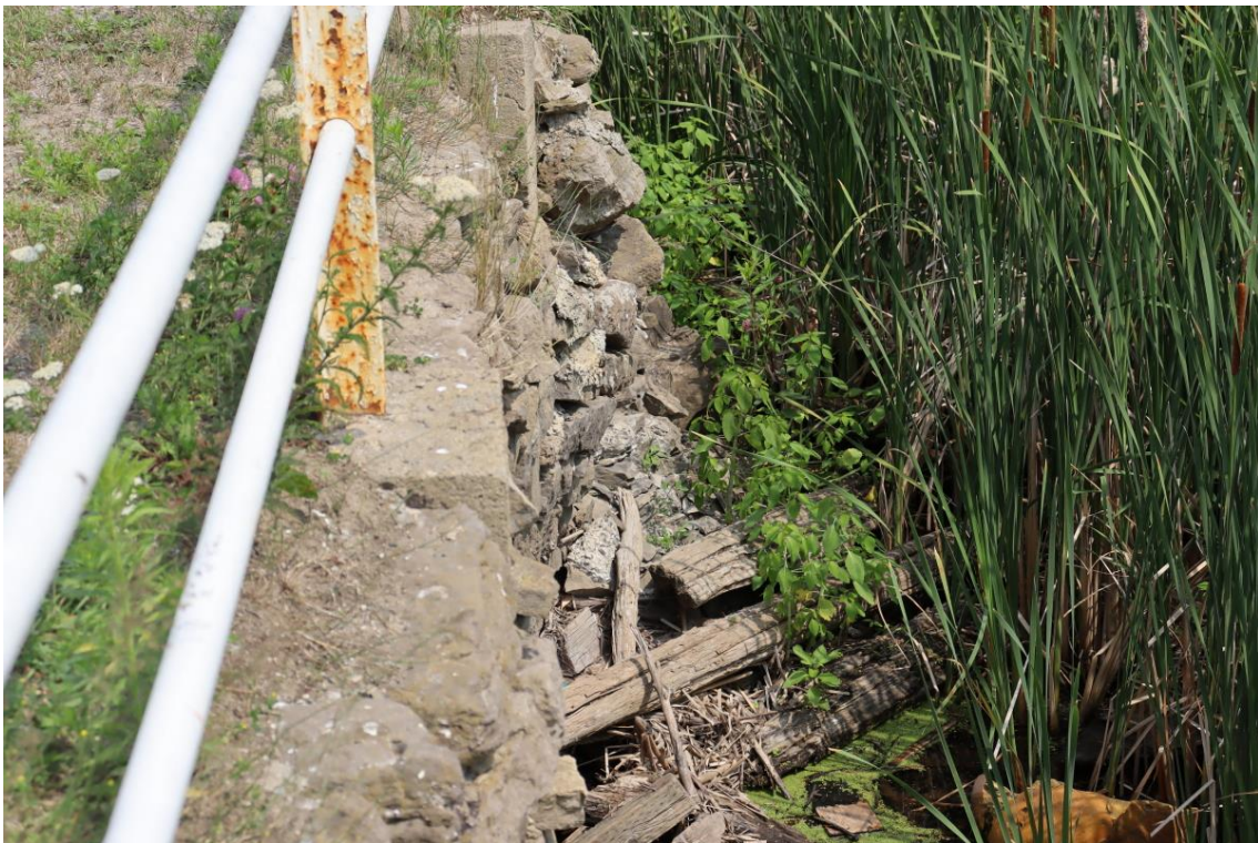
Figure 32: Bulging retaining wall in SE
