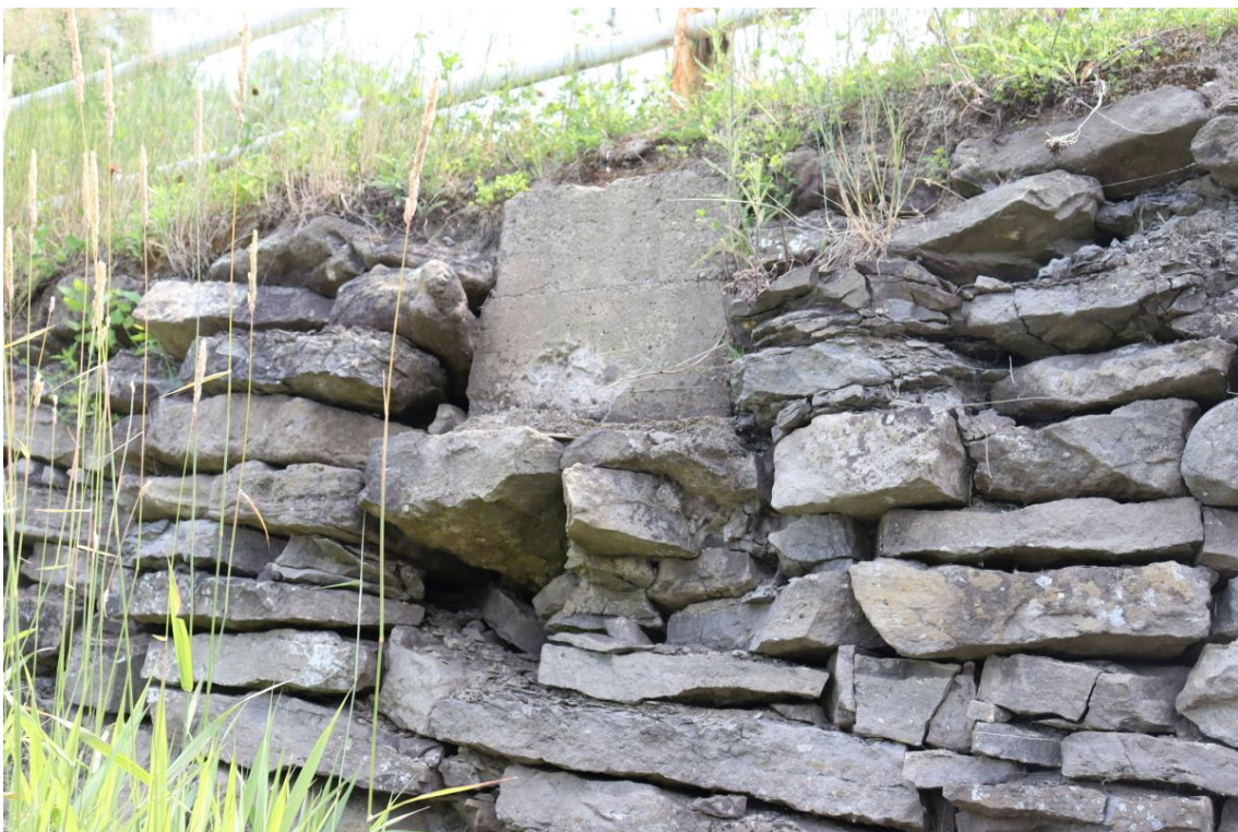
Figure 50: North-east quadrant dry-stone retaining wall
