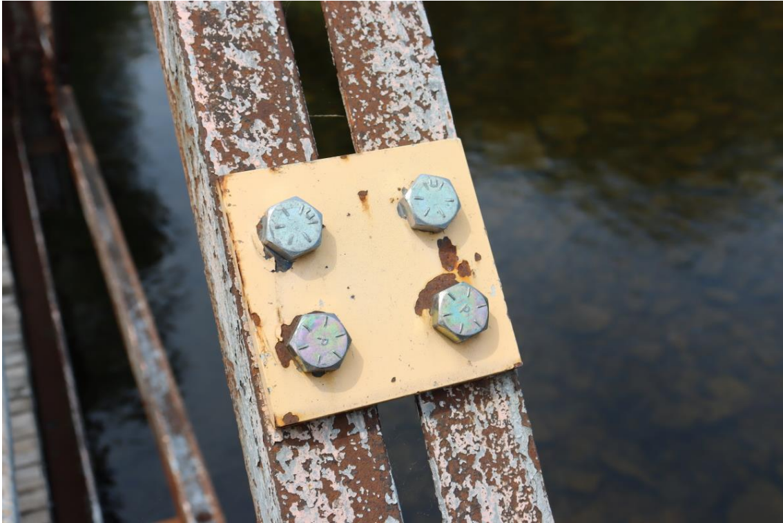
Figure 59: Typical compression diagonal bracing tie plate
