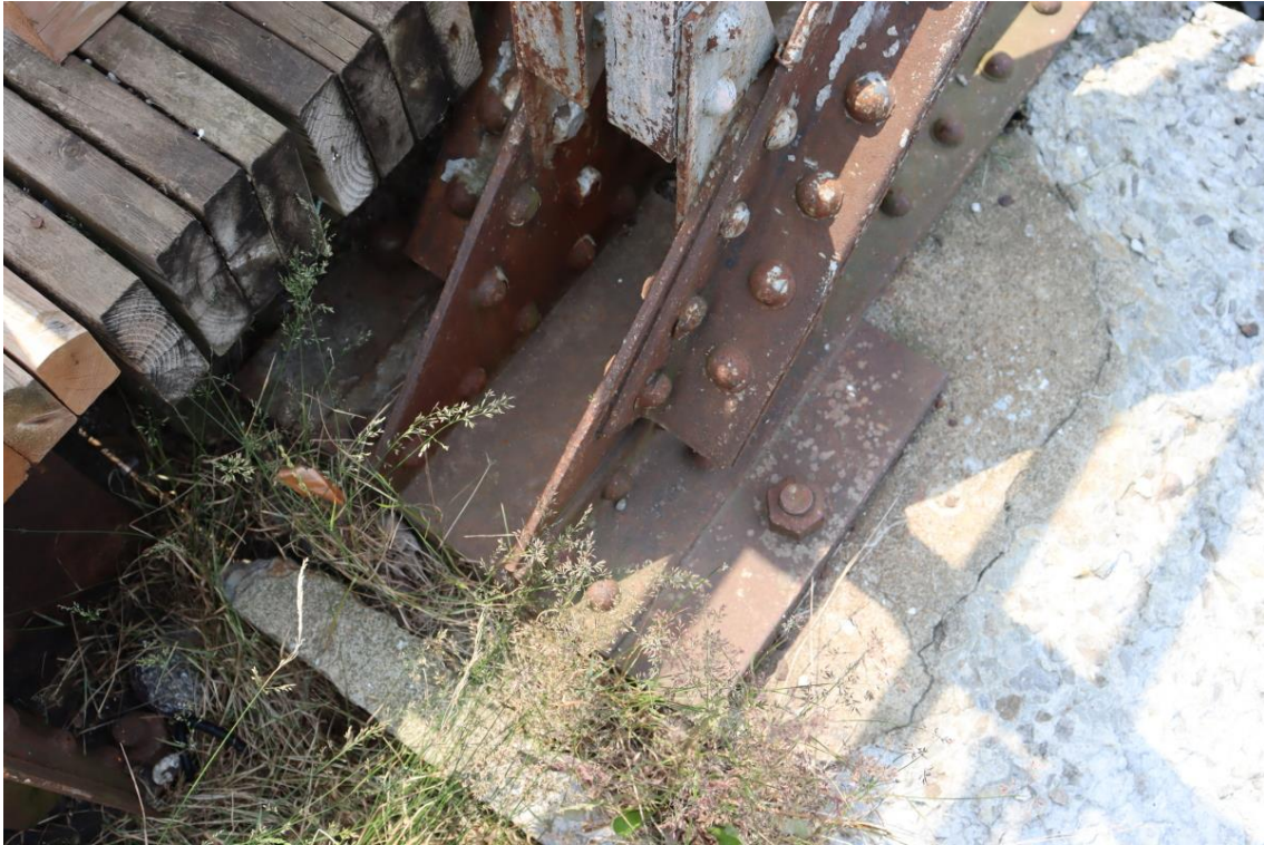
Figure 45: North pier truss bearing
