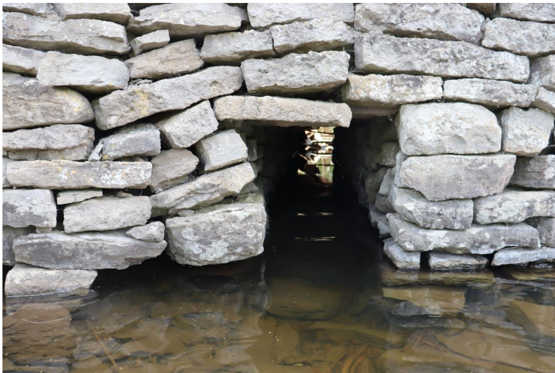
Figure 51: Drainage opening through causeway
