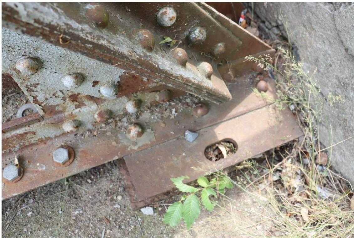
Figure 33: NW truss bearing
