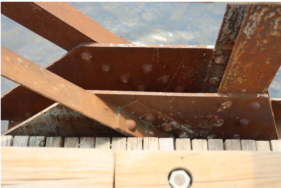
Figure 56: Typical bottom chord connection
