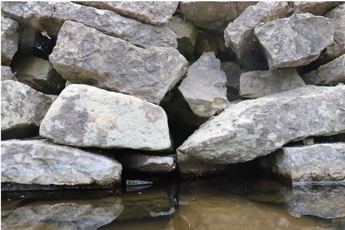
Figure 49: Blocked drainage opening through causeway
