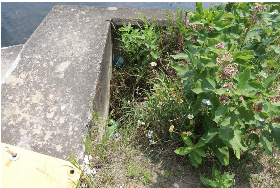
Figure 42: Sinkhole in SW corner
