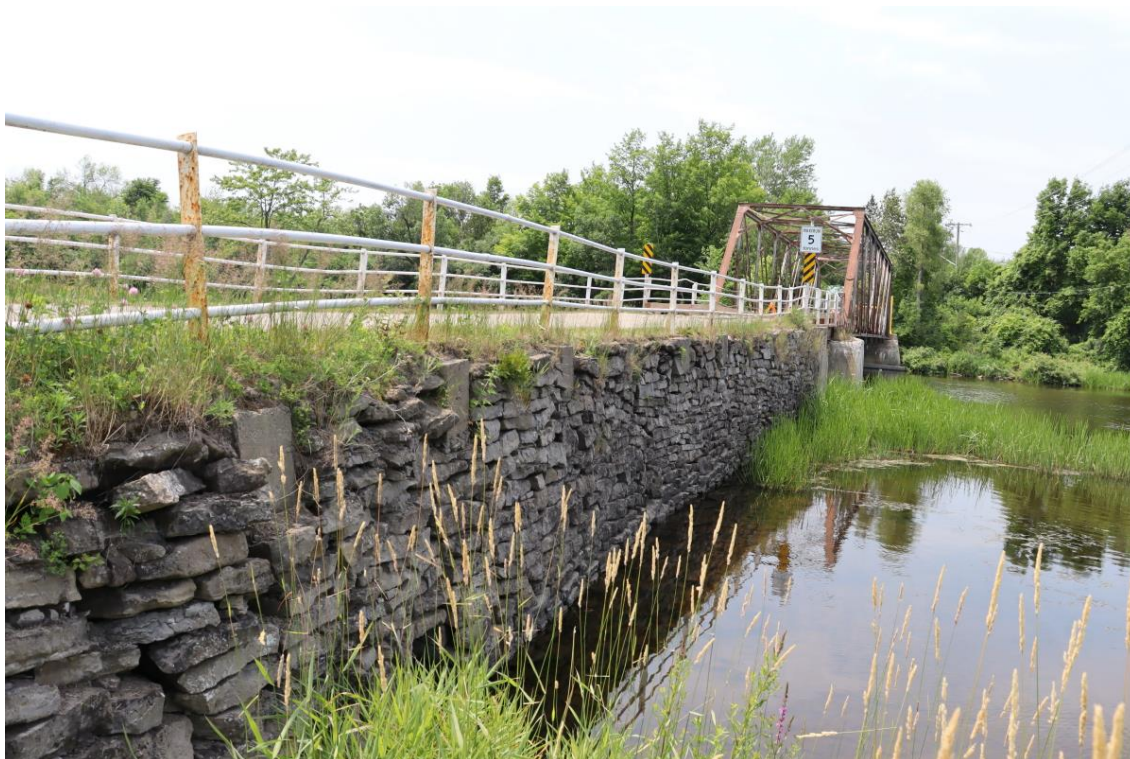
Figure 53: North dry-stone retaining wall east approach
