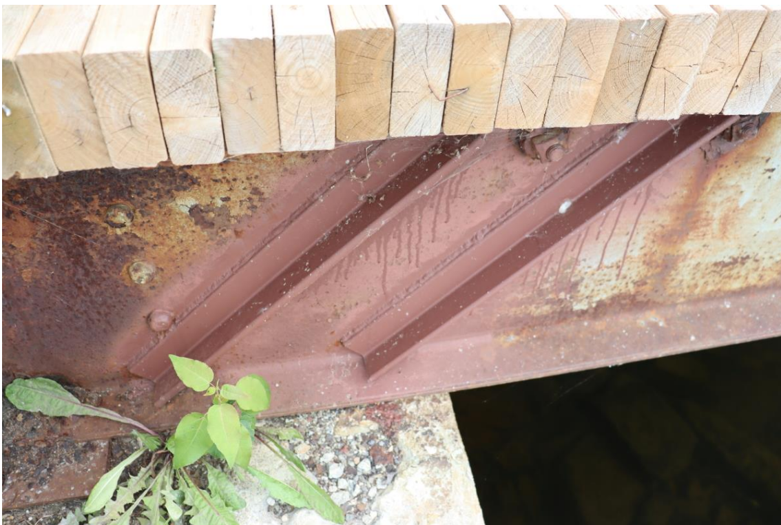
Figure 26: NE girder end web stiffening
