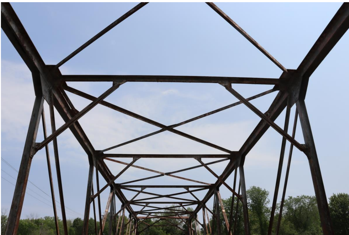
Figure 64: Wind and sway bracing
