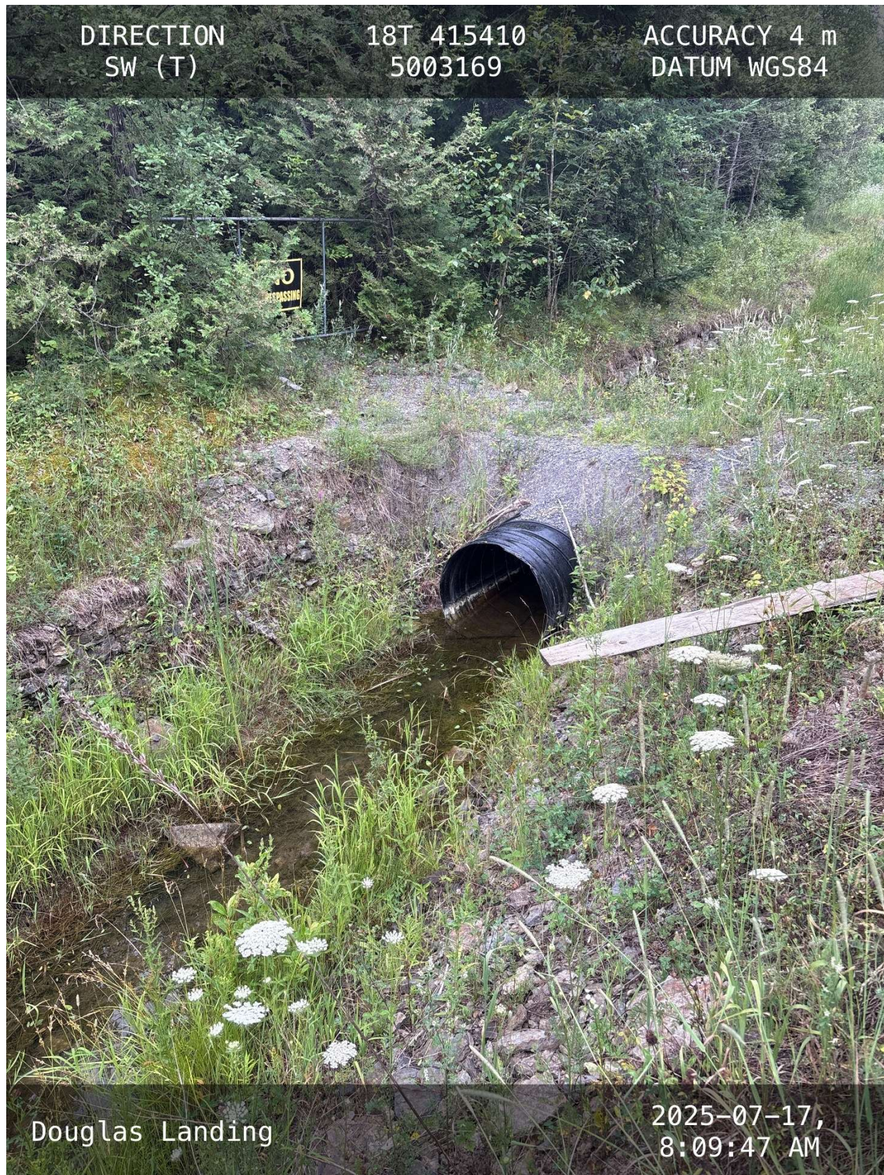
Photo 6: Steel Culvert and Gravel Berm, MMD2, July 2025
