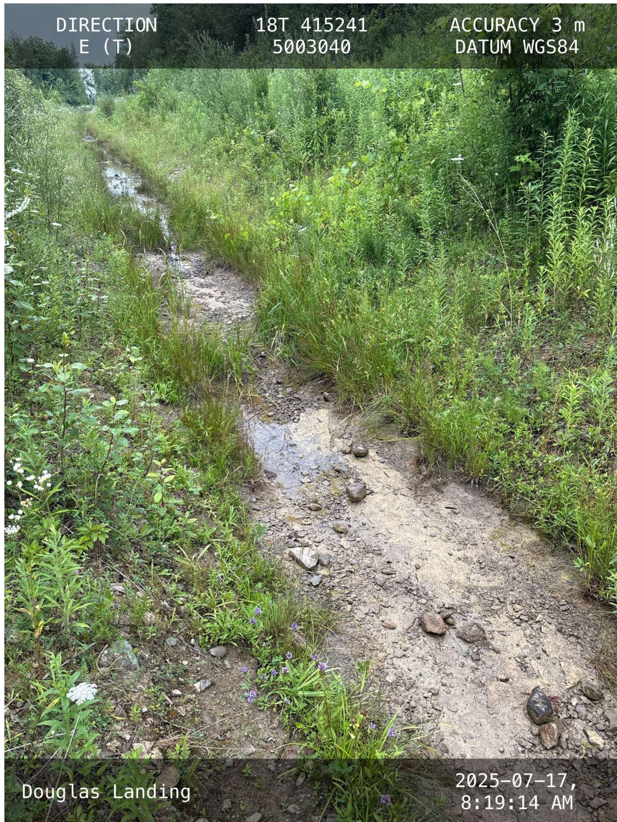
Photo 8: Downstream Extent of Wetted Channel, MMD2, July 2025
